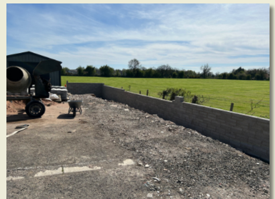
Retaining Wall on Perimeter
